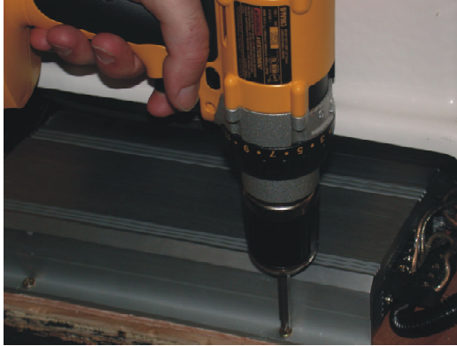
Figure 51. Securing Amplifier to the Frame
